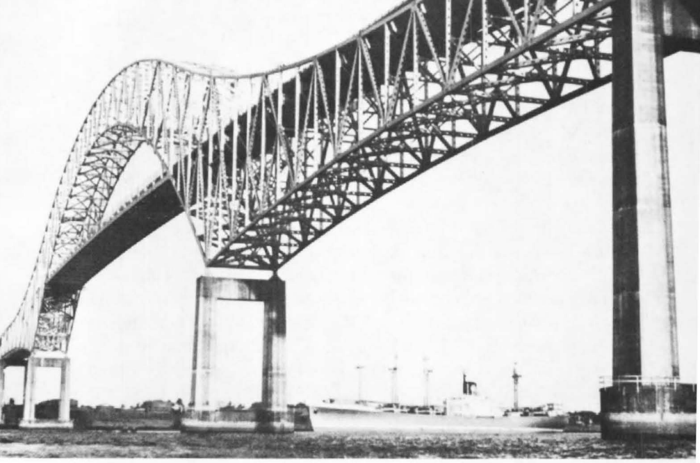
Thatcher Bridge over Panama Canal Courtesy Pan American Union
